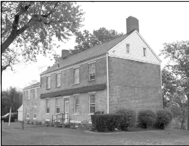
The historic Van Veghten House sits on a bluff above the floodplain. Credit: Lynn Rakos, Archaeologist, New York District, U.S. Army Corps of Engineers.
