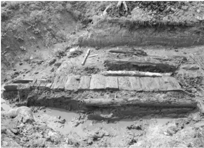
Culvert, possibly from 17th-century road construction through dyked marsh lands at Grand Pré. Photo: Rob Ferguson, Parks Canada.
