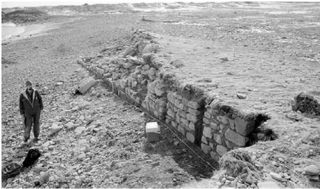
French curtain wall exposed by winter storm. Photo: Rebecca Duggan, Parks Canada.
